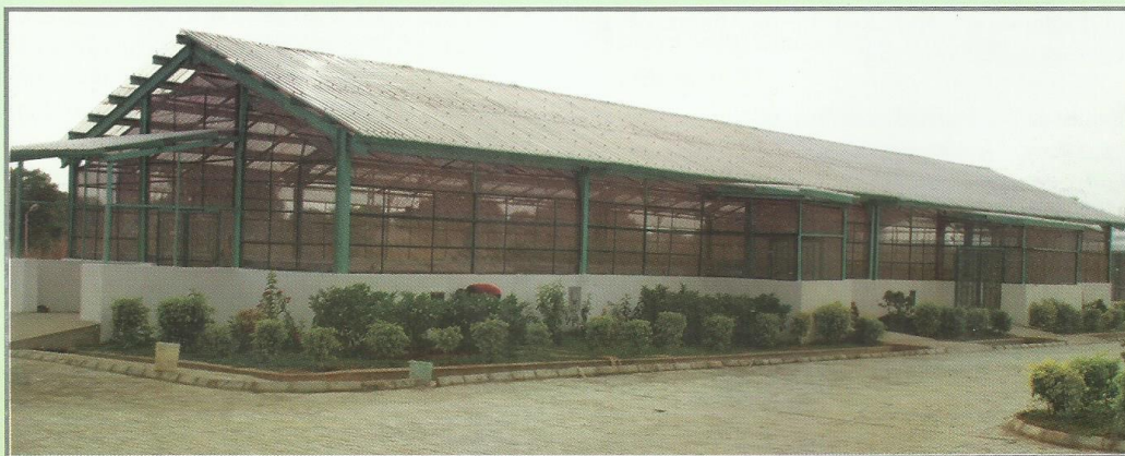
Green House at the Bio-Factory Site
